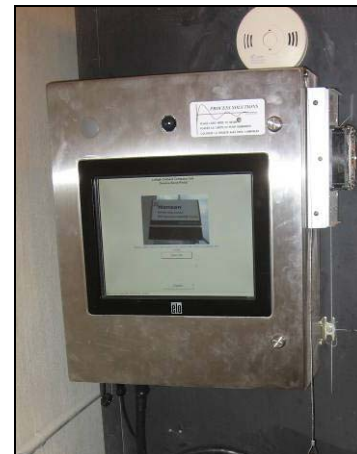
Plant Portal Kiosk
